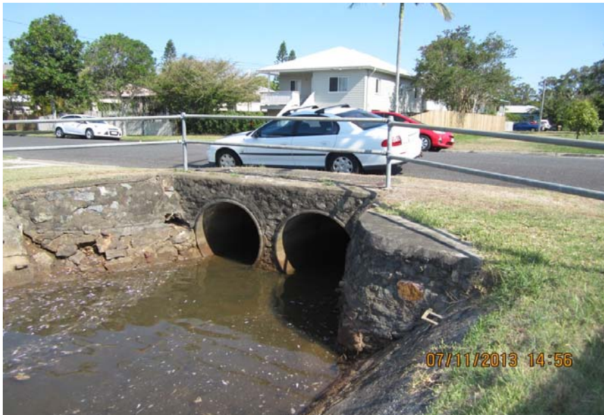
Queens ParadeSouth culvert -Downstream view at Seaview Street crossing
