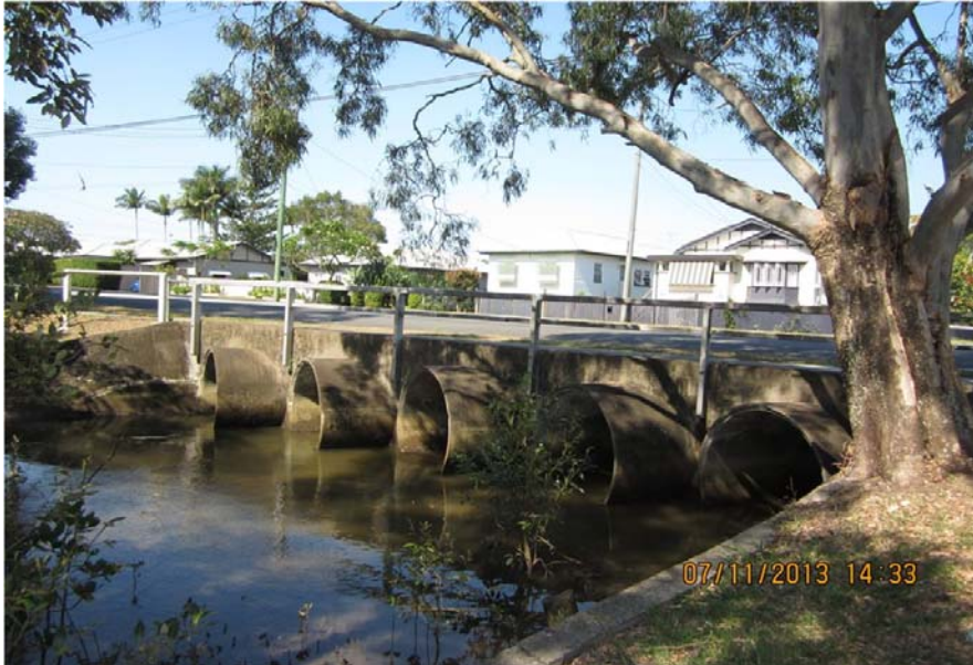
Beaconsfield Terrace culvert looking downstream
