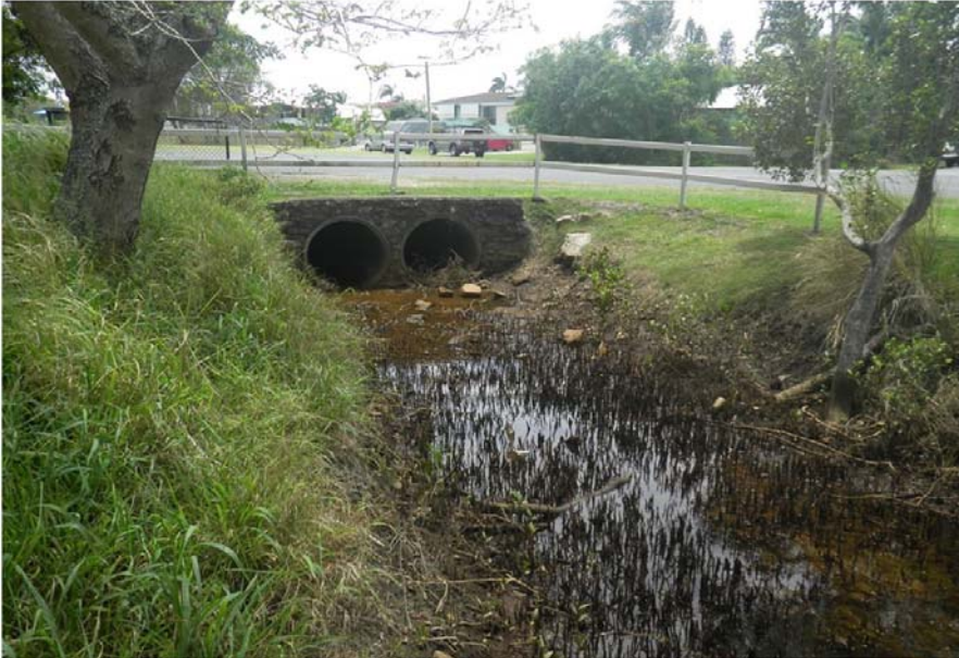
Queens Parade culvert South looking downstream
