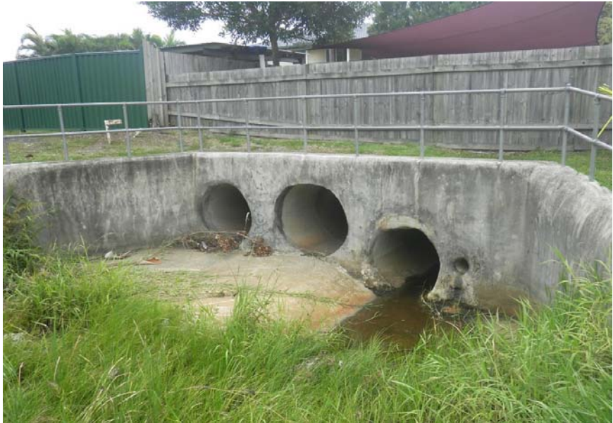
Wickham Street culvert looking downstream
