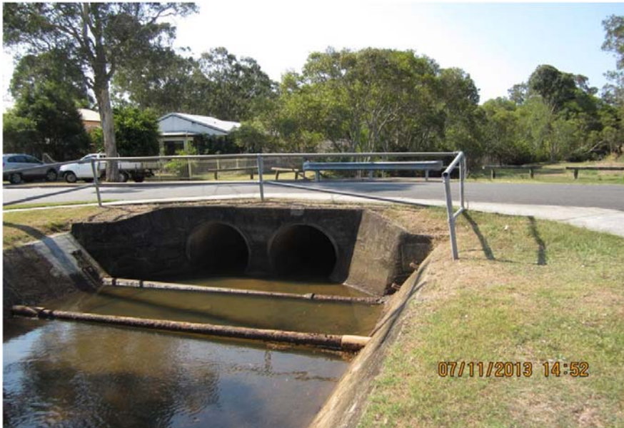
Townsend Street culvert looking downstream
