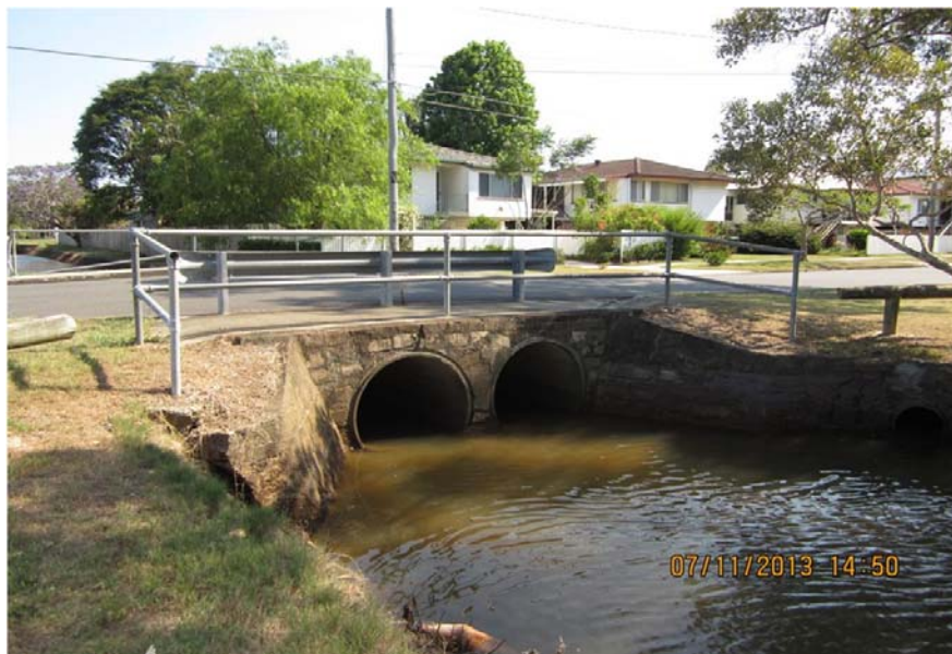
Townsend Street culvert looking upstream
