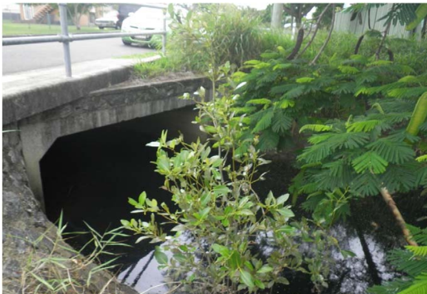
Shepherd Street culvert looking upstream
