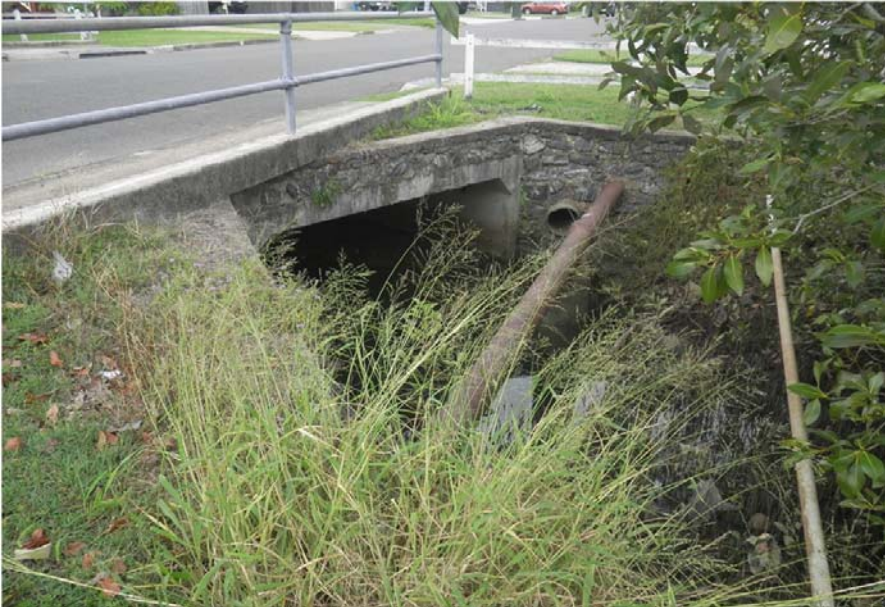
Shepherd Street culvert looking downstream
