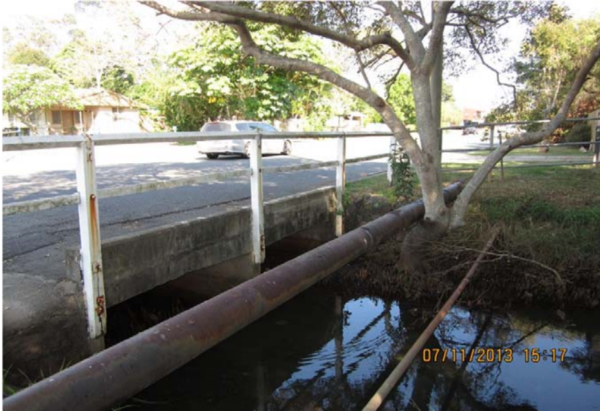
Queens Parade culvert North looking downstream
