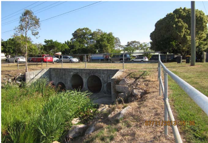
Wickham Street culvert looking upstream
