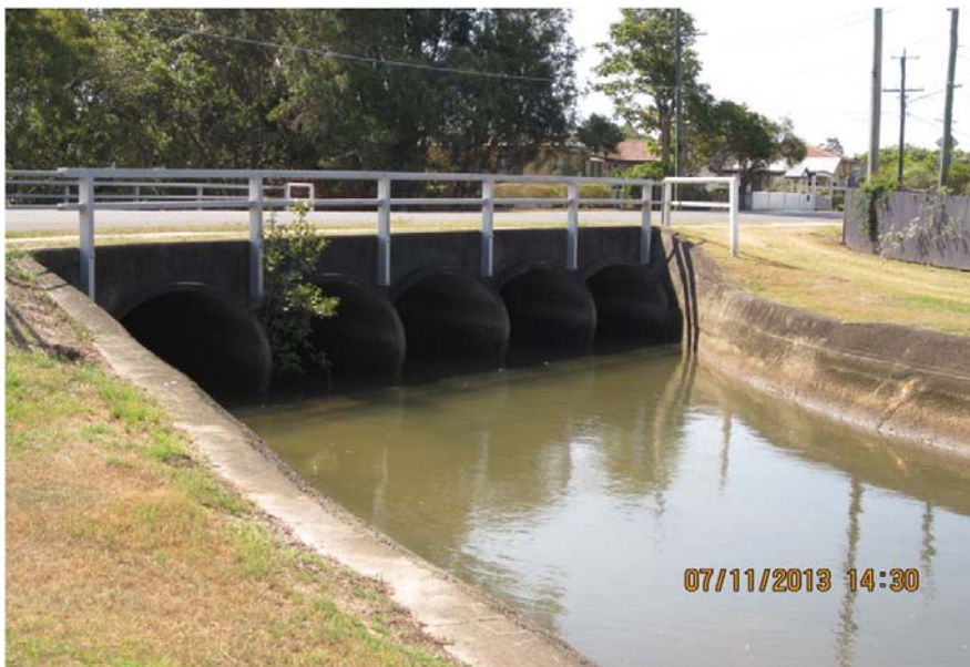
Beaconsfield Terrace culvert looking upstream
